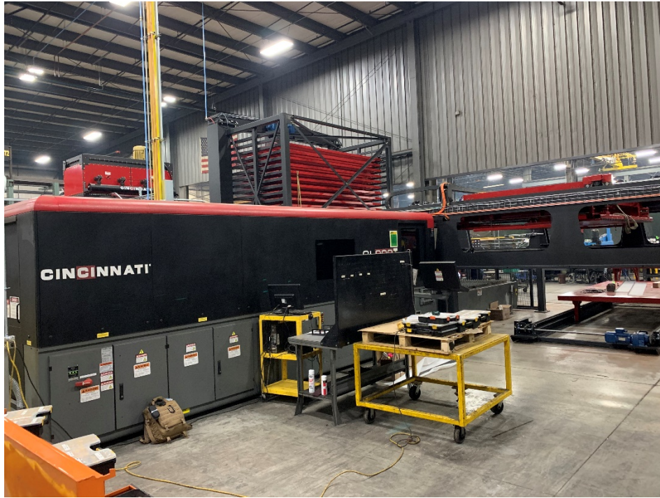
Mega Fab Robotic Material Handling system seen from a distance which feeds the laser in the foreground.
